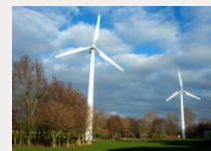
Wind Turbines, GSK Barnard Castle
