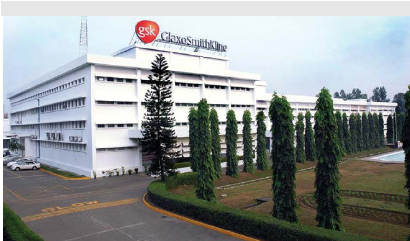
A view of manufacturing site of GSK Bangladesh in Chittagong
