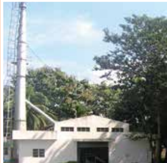
Effluent Treatment Plant (ETP) at GSK Chittagong Site
